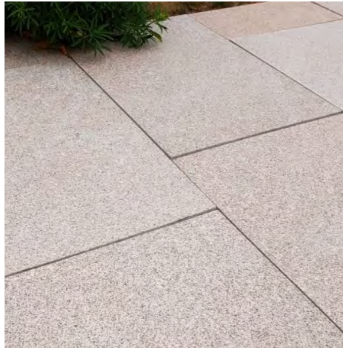
Paving Type 22: Buff Coloured Granite Slabs Size: 600x600mm, depth 50mm. Colour: 3 shades of light buff. Supplier: Stonepave or Similar Approved
