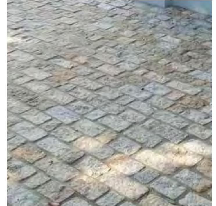
Paving Type 20: Buff Coloured Granite Setts Size: 100x200, depth 50mm. Colour: 3 shades of light buff. Supplier: Stonepave or Similar Approved
