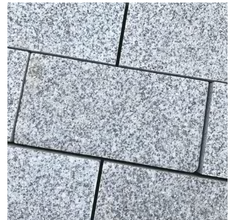
Paving Type 8: Buff Coloured Granite Setts Size/Colour 100x200, depth 80mm / to meet DCC standards. Supplier: Stonepave or Similar Approved
